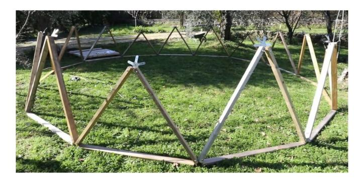
Once again, it's important to support these triangles until the belt is assembled using other temporary struts:
