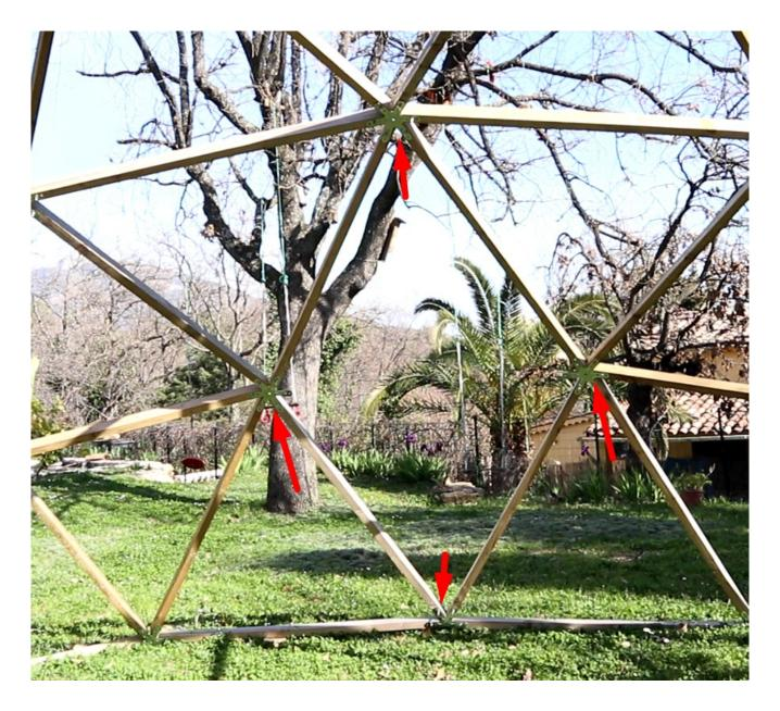
In these cases, I advise you to reinforce the structure by adding wood screws in each free hole of the 4 connectors around your new opening.
