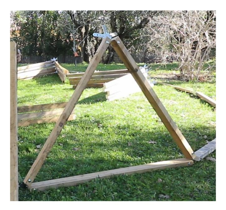
IMPORTANT: I advise you to add a support on these triangles as long as the belt is not installed. Use temporary struts to support these triangles.
