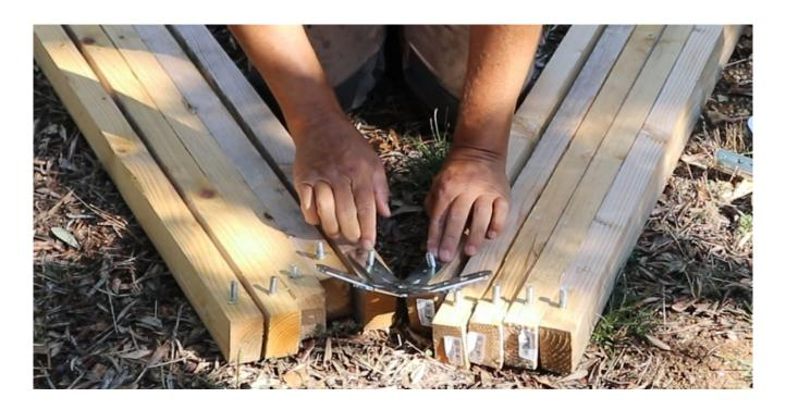
Place these triangles on the base between 2 **large-hole** legs (NOTE: the concave side towards the ground!)
