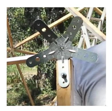
Screw this upright (with the C5 connector) into one of the connectors on the high belt from step 6
