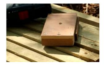
Now complete the 130 holes (!) in the studs using your template and trying to drill as straight as possible
