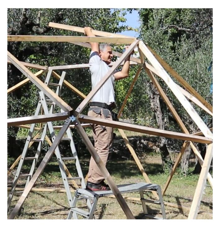
Add the other uprights, attaching them each time to the high belt and to the last C5 connector installed at the top
