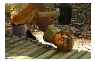
**Tip**: if the hammer isn't enough, you can use a screw and washer and tighten the bolt so that it goes into the wood
