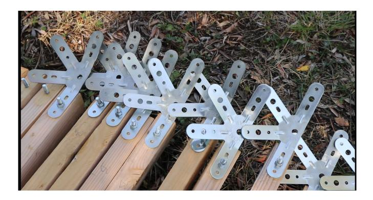
Taking care to separate the 4.1 and 4.2 connectors, screw the left-hand leg of the 10 connectors into a large B-post
