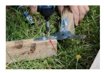
Here are the sets of 3 uprights ready to be fitted (unlike this image, remember to use 2 wood screws per branch):
