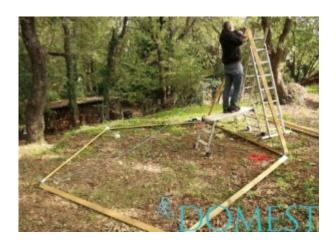
• Tighten and tie the cord: the top of the triangle should extend a little beyond the base (the projection of the top of the triangle should be a little outside the base). This cord should support the triangle throughout the assembly of the walls and the high belt.
