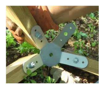
■ Take a new upright without a connector and bolt / screw it to the next 4-branch connector on the base to form a triangle while supporting the top on the ladder
