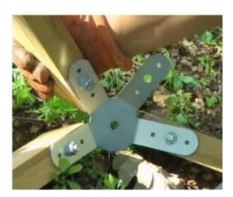
■ Take a new upright without a connector and bolt / screw it to the next 4-branch connector on the base to form a
