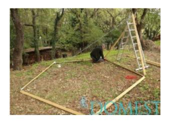
• Finish the triangle by screwing / bolting the top of the triangle.
