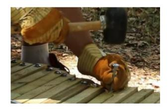
**Tip:** If the hammer is not enough you can use a screw and washer and tighten the bolt so that it goes into the wood.
