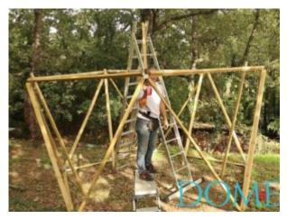
Repeat for the other 4 posts Now assemble all the posts at the top of the geodesic dome.
