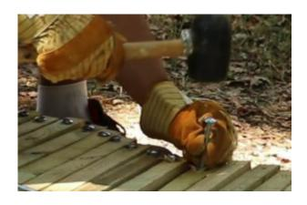
**Tip**: If the hammer is not enough you can use a screw and washer and tighten the bolt so that it goes into the wood.
