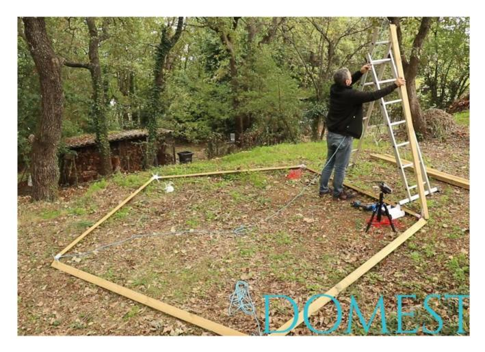
Screw / bolt the upright to an inner leg of a 4-branch connector of the base. For this operation you can get help from a person holding the upright or from a ladder that will hold the upright while you screw / bolt. This new upright must be supported while screwing.
