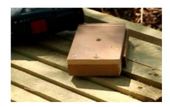
Now finish the holes in the uprights, using your template and trying to drill as straight as possible.
