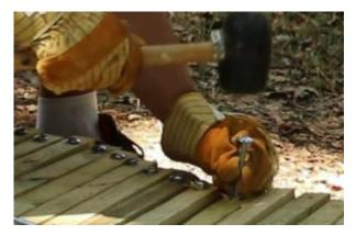
**Tip**: if the hammer isn't enough, you can use a screw and washer and tighten the bolt so that it goes into the wood.
