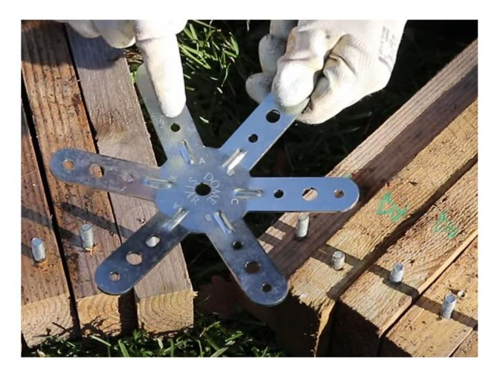
Now assemble the last 5 pairs with the 6Ms, but this time with B on your right and A on your left. The letter X on the 6M connector will be on your left.
