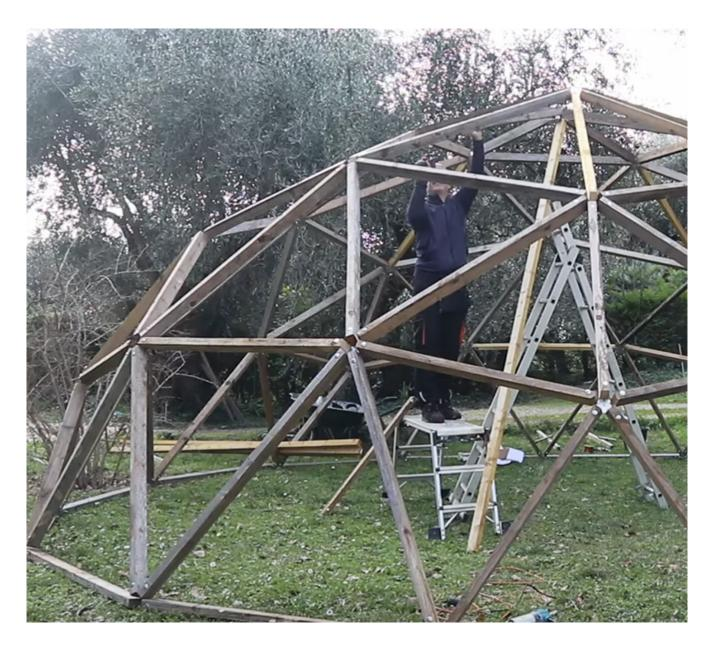
I install the 4 missing connectors by screwing them on.
