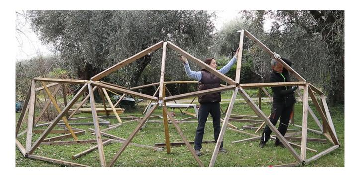
immediately attach the belt strut connecting the first 2 triangles
