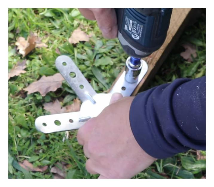
I screw this upright onto the dome. It needs to be supported while the other connectors are installed.
