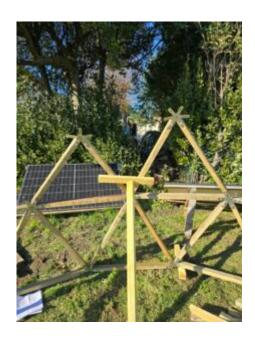
Here too, it's important to support these triangles until the belt is fitted using other temporary uprights.
