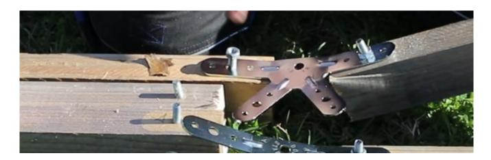
Finally, assemble the base to the floor, alternating our two types of uprights.
