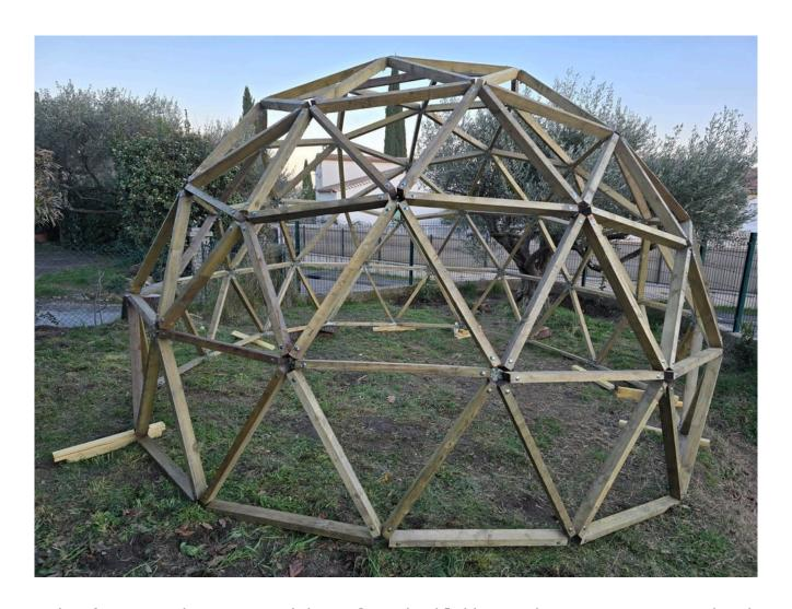
I don't yet have a video for building the 3V 5/8 geodesic dome, but you can watch the video for building the 3V 3/8 dome. However, in this old video I put up all the triangles of a floor before putting on the belt of this floor: I do NOT recommend this way of doing things. I recommend putting the belt on as the triangles are assembled.
