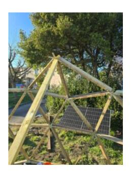
And we'll continue circling the dome, installing the 2-leg and 3-leg triangles in turn and, above all, gradually adding the 3rd belt made up exclusively of A-pillars:
