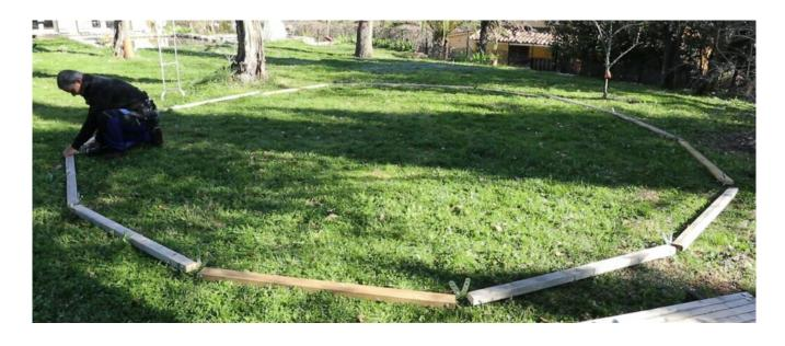
Once your base is assembled, you can roughly check the lengths of a few diagonals to make sure you haven't made an oval. There's no need to be centimetre accurate here, but if you have a 1 metre difference in your diagonals you'll struggle later! Everything adjusts itself during assembly, but with varying degrees of effort!
