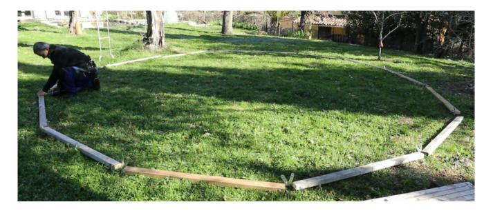
Once your base is assembled, you can roughly check the lengths of a few diagonals to make sure you haven't made an oval. There's no need to be centimetre accurate here, but if you have a 1 metre difference in your diagonals you'll struggle later! Everything adjusts itself during assembly, but with varying degrees of effort!
