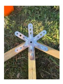
Equipped with your 3-leg triangles, be careful: the central leg B must be fitted to a 6M connector, not 6A.
